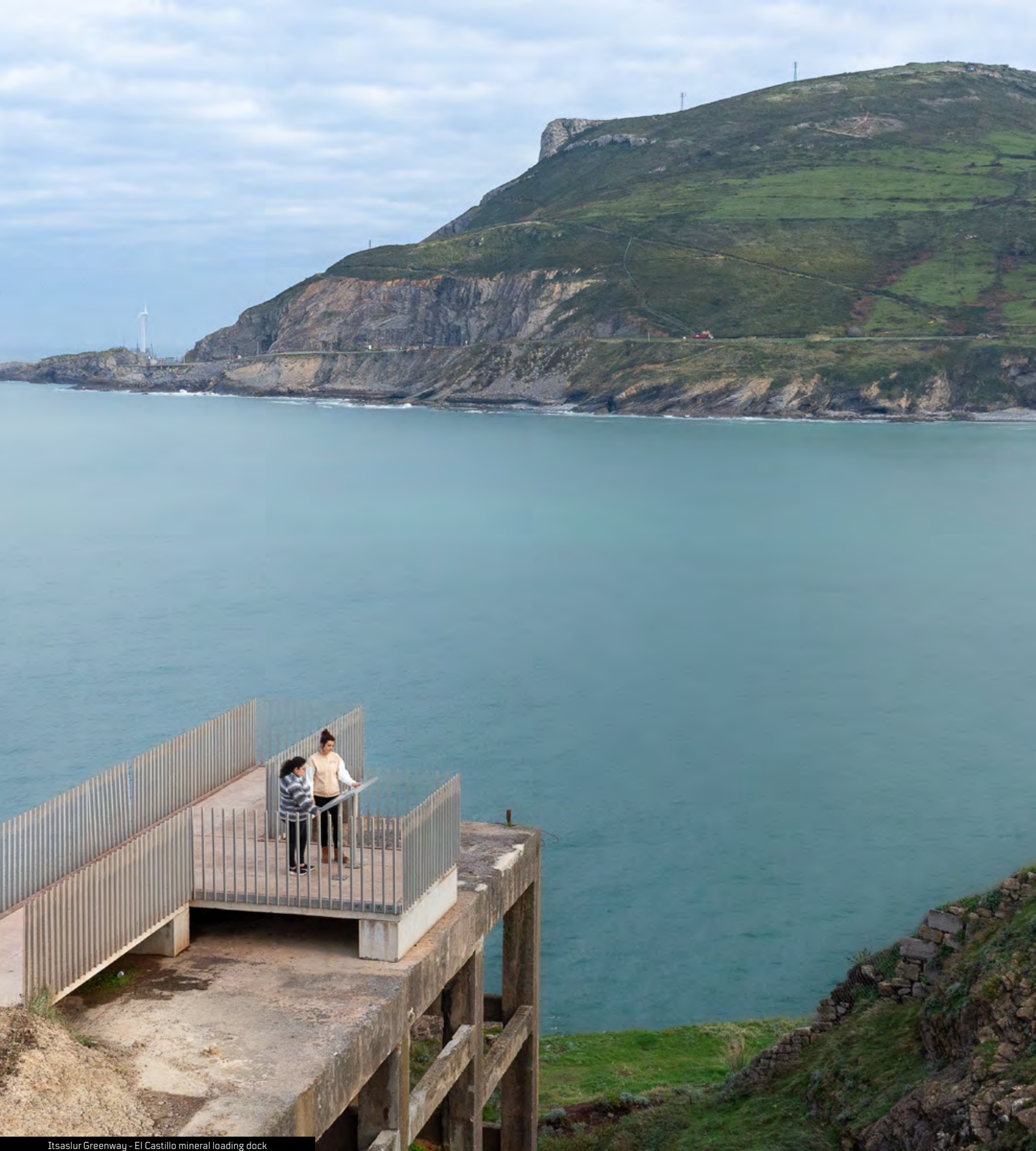
Itsaslur Greenway - El Castillo mineral loading dock
