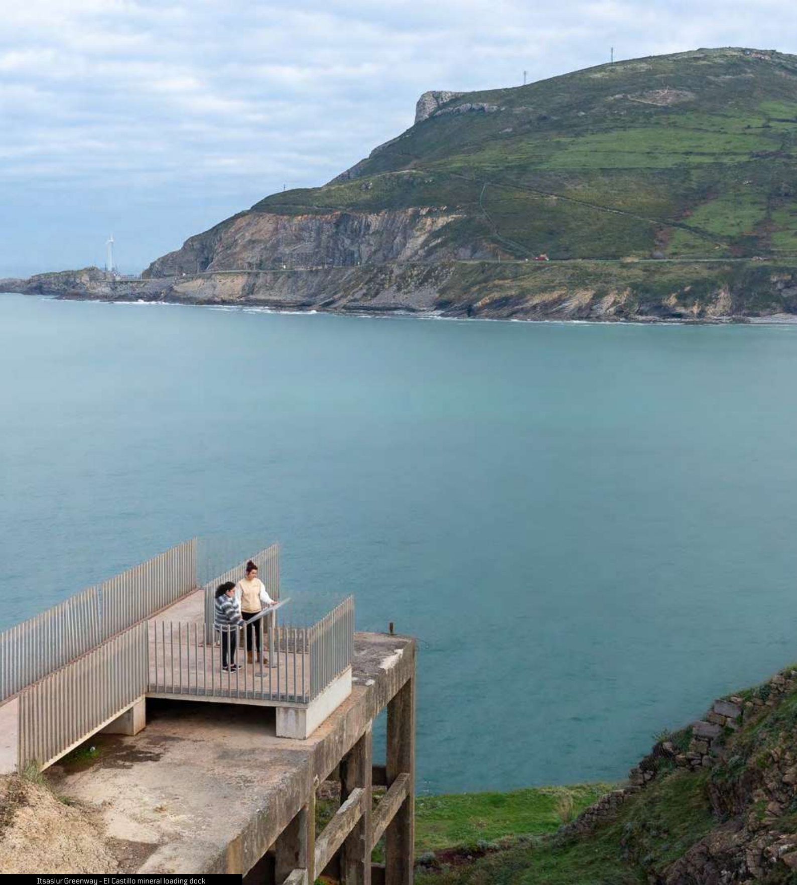
Itsaslur Greenway - El Castillo mineral loading dock
