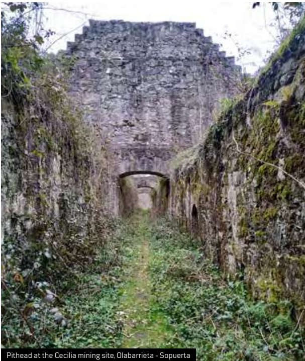
Pithead at the Cecilia mining site, Olabarrieta - Sopuerta
